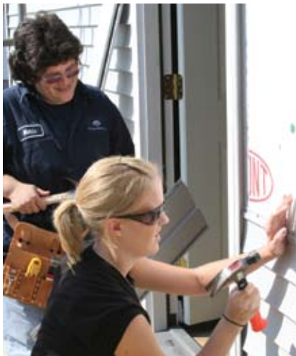
Employees help build Habitat for Humanity homes near our Global Headquarters.
